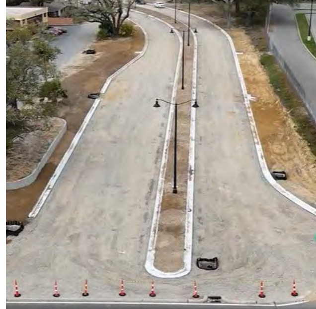
Popp's Ferry Extension roadway taking shape
