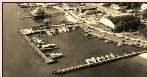
↳ The USO building (upper right of photo) was designed and positioned to take advantage of its waterfront location, with a 100 ft by 14 ft screened porch overlooking the small craft harbor and the Mississippi Sound. The Biloxi Yacht club is seen in upper left of photo. Source: Keesler News .
