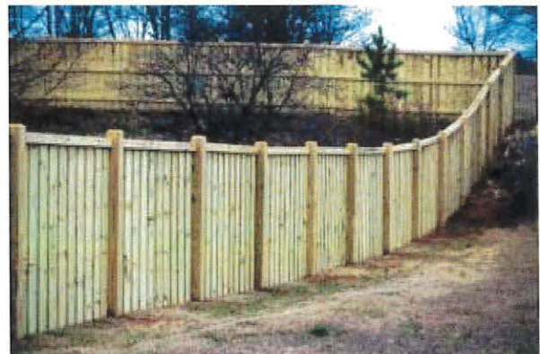
Figure 23-6-7(F)(1): Fence with Finished Side Out
