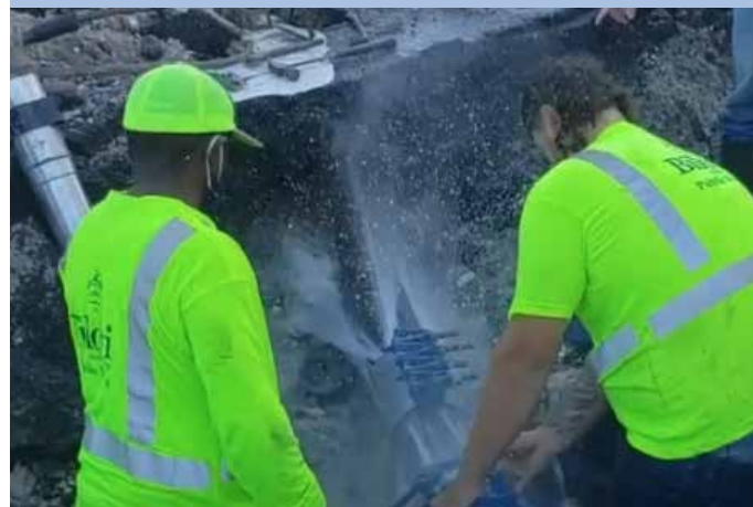
Public Works crew repair water main break at G E Ohr and U.S. 90
