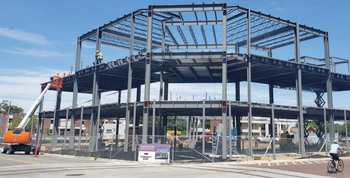
Construction workers hang steel on the new Community Bank building in downtown Biloxi.
