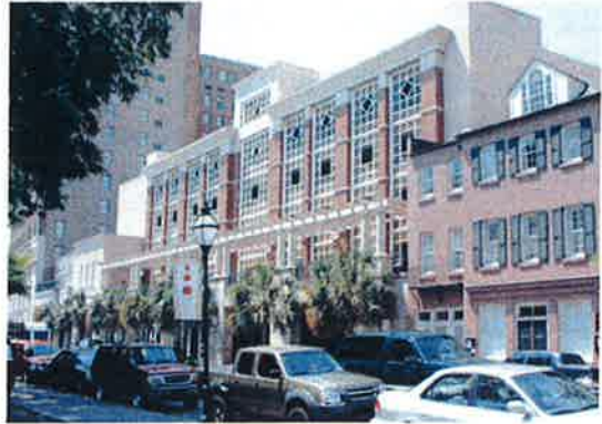
FRANCIS MARION HOTEL PARKING GARAGE – CHARLESTON, SC
