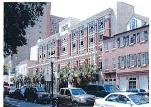
FRANCIS MARION HOTEL PARKING GARAGE – CHARLESTON, SC
