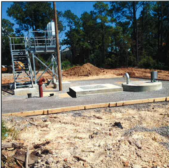
NOB4- Bayside East Pump Station
