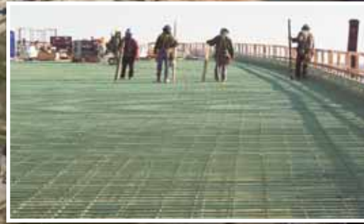
Workers check the section of rebar
