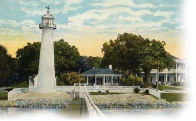
The design of the Biloxi Lighthouse called for a structural system of cast iron plating with an inner lining of brick for strength and stability. Only one cast iron lighthouse had been built in America, and some people thought the plan to use this relatively new material was risky.
