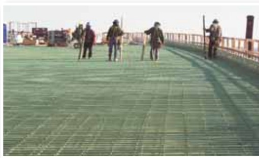
Workers check the section of rebar months ago.
