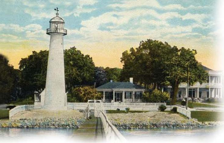
The design of the Biloxi Lighthouse called for a structural system of cast iron plating with an inner lining of brick for strength and stability. Only one cast iron lighthouse had been built in America, and some people thought the plan to use this relatively new material was risky.
