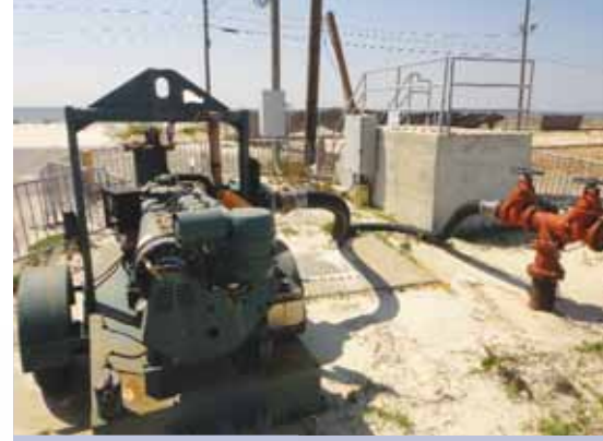
Bypass pumps were put into service where Katrina's storm surge destroyed the electrical panels and pumps that drove the pump stations. Note the elevated platform in the background of the photo. Obvious question: So why are these pump stations placed in harm's way, so near the Biloxi beach? In order to be effective, they must be situated at or near the lowest point. The city is reducing the number of pumping stations and hardening those that must remain in harm's way.
