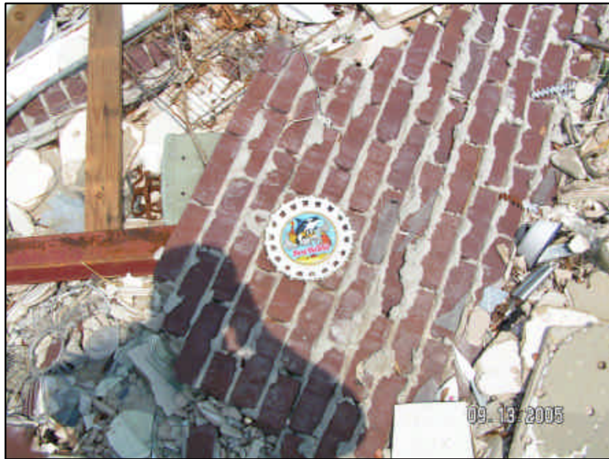
Ironically, despite the destruction of everything around it, a porcelain commemorative plate is found on the remains of a wall at Beauvoir Beach in mint condition.
