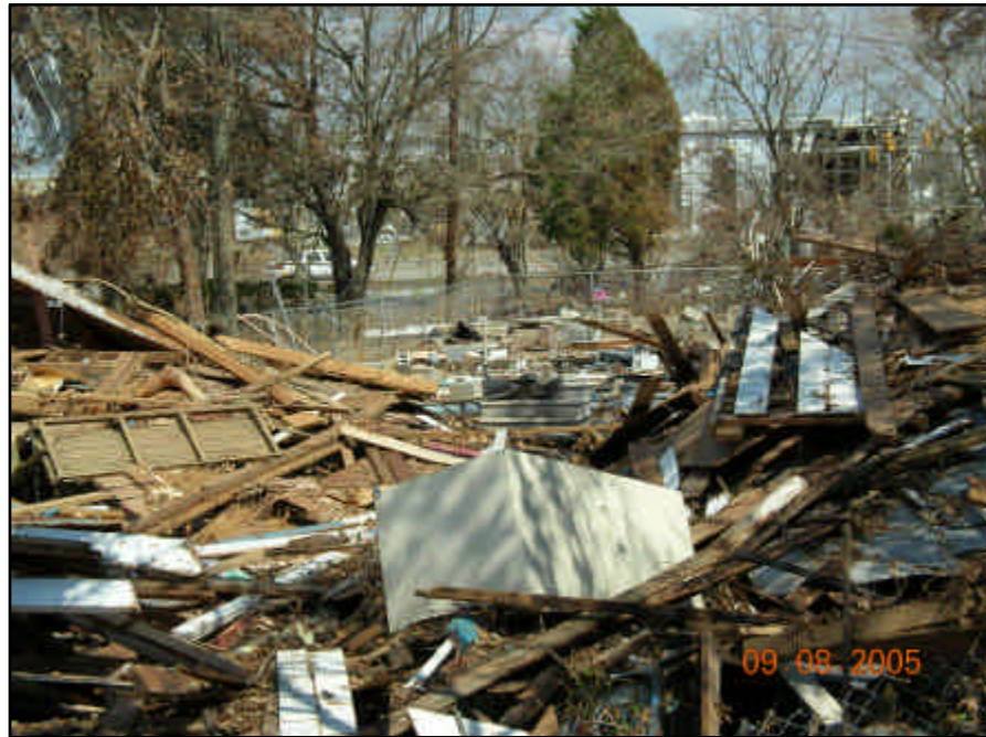
Debris floated onto the HOPE VI project site.
