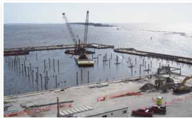
New moorings are installed at the Biloxi Small Craft Harbor.
