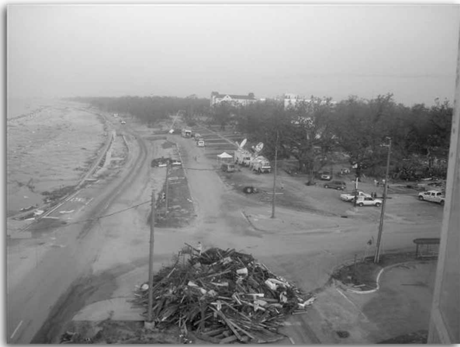
Workers had cleared sections of U.S. 90, as seen from atop the Biloxi Lighthouse.
